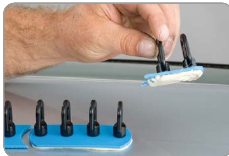
Place the pad firmly to the surface, let the glue cool down.
